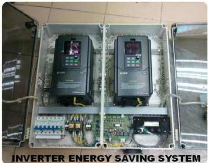
RPM & TEMPERATURE CONTROL SYSTEM
